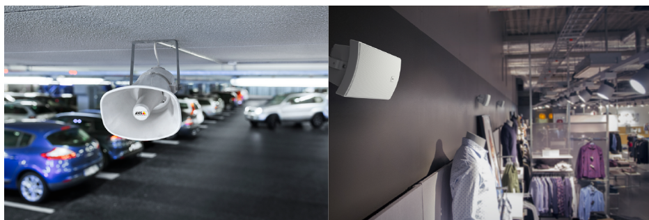
Figure 1.3a Network audio can be installed for security or safety purposes, or for operational efficiency.
